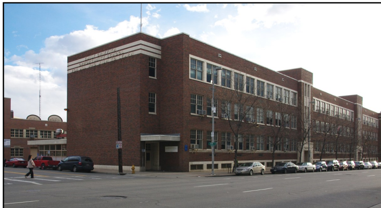
5. View of the school from Welton and 13th Streets. The historic structure conveys its massing, volume and form as a distinct entity.
