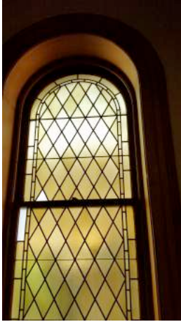
Original stained glass window
