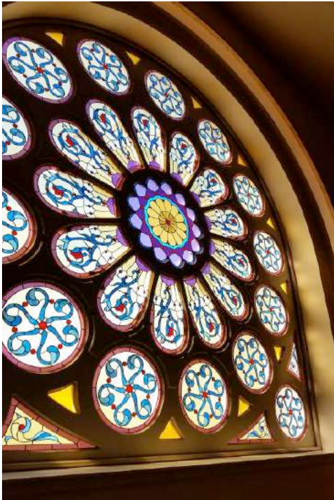
Watkins Rose Window on South Wall
