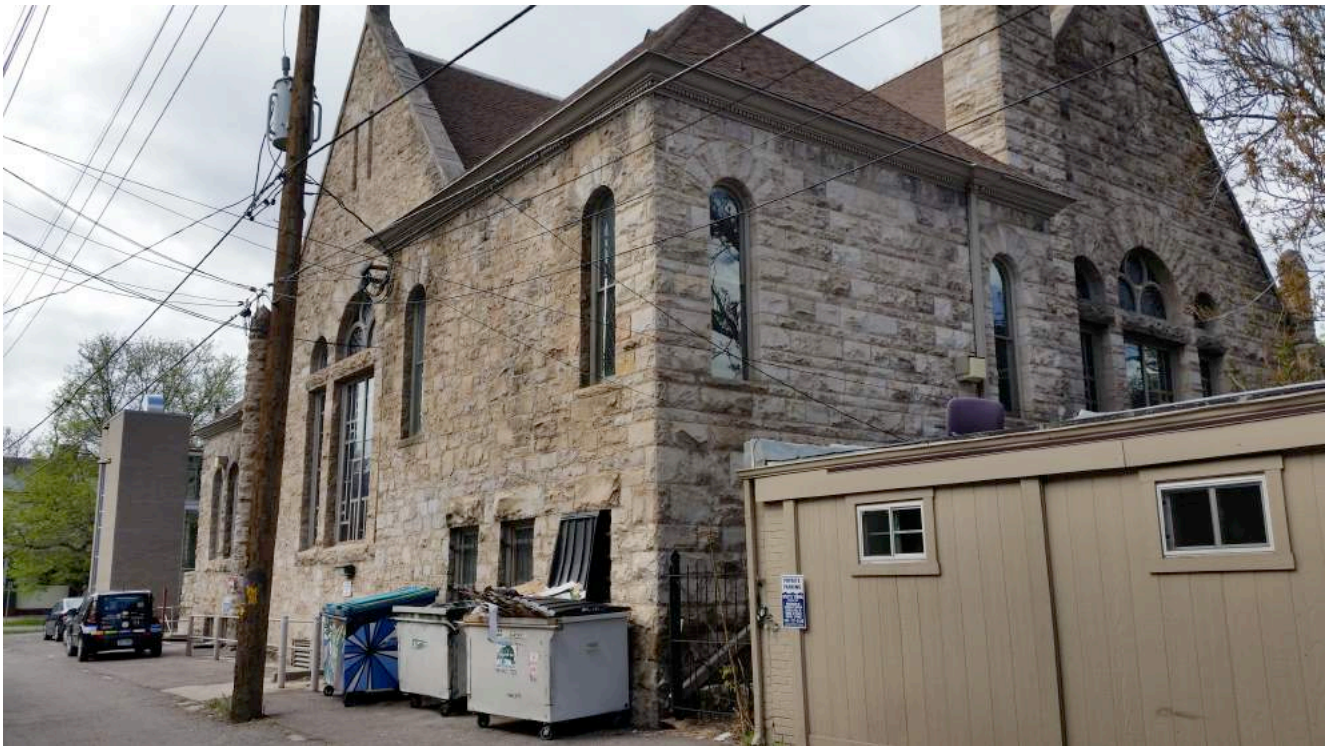
First Unitarian Society of Denver: Northeast Corner
