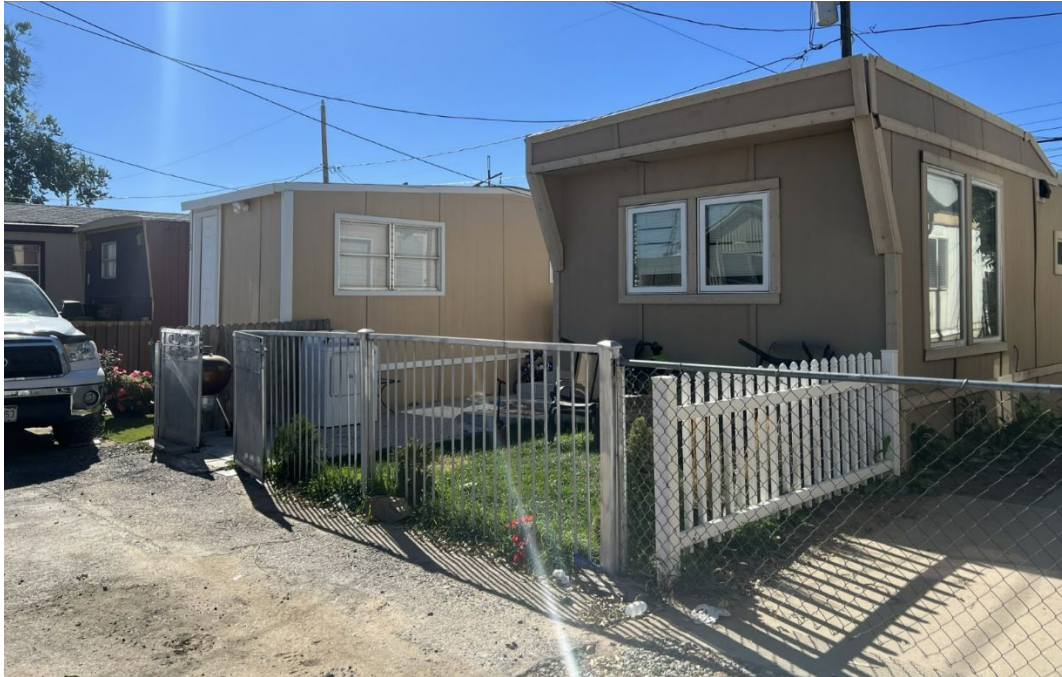
View of mobile home park at 5220 Steele Street and 5201 Adams Street in District 9.
