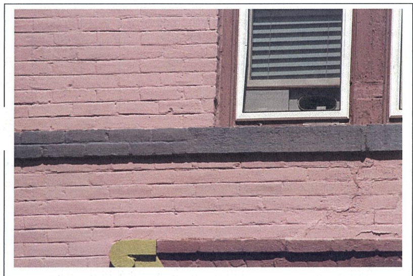
8. Painted belt course and stone sill detail
