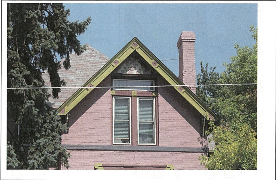
3. South elevation - upper wall detail
