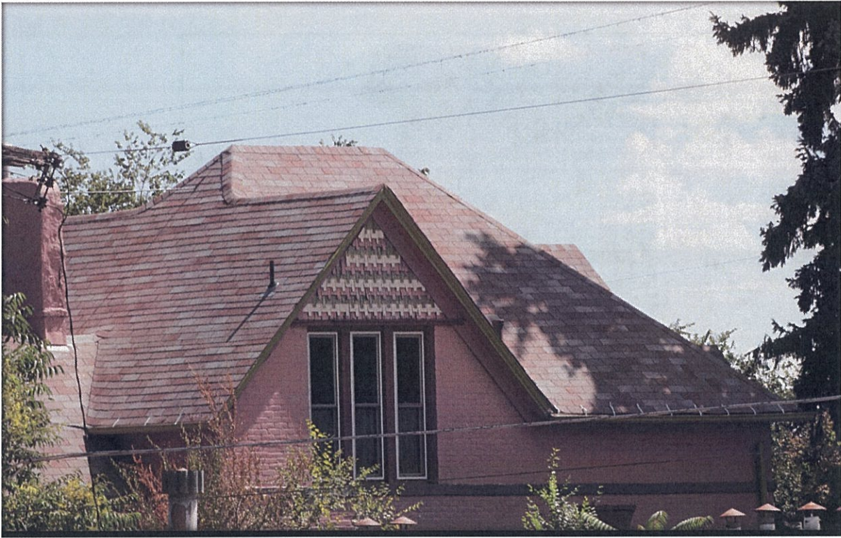
11. View of Upper West Elevation
