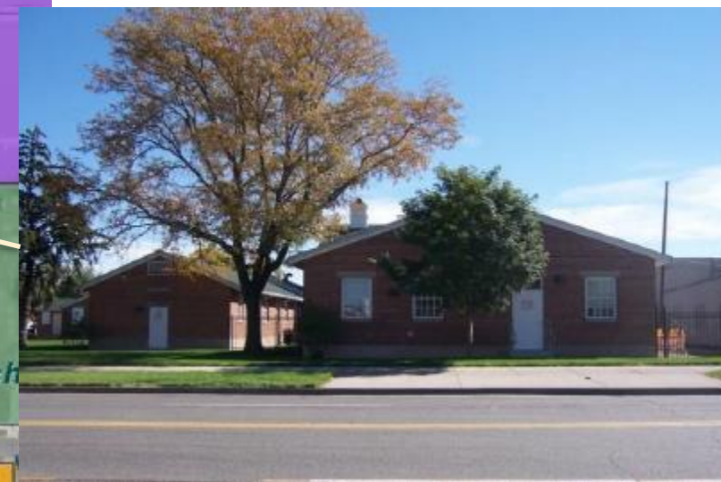
Inner City Health Center looking east
