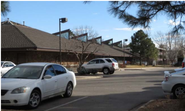
Office Building on subject site.
