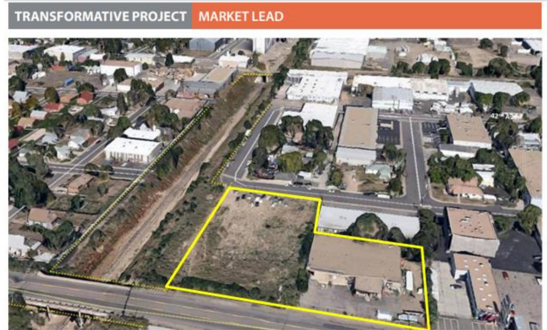
Market Lead underpass existing condition
