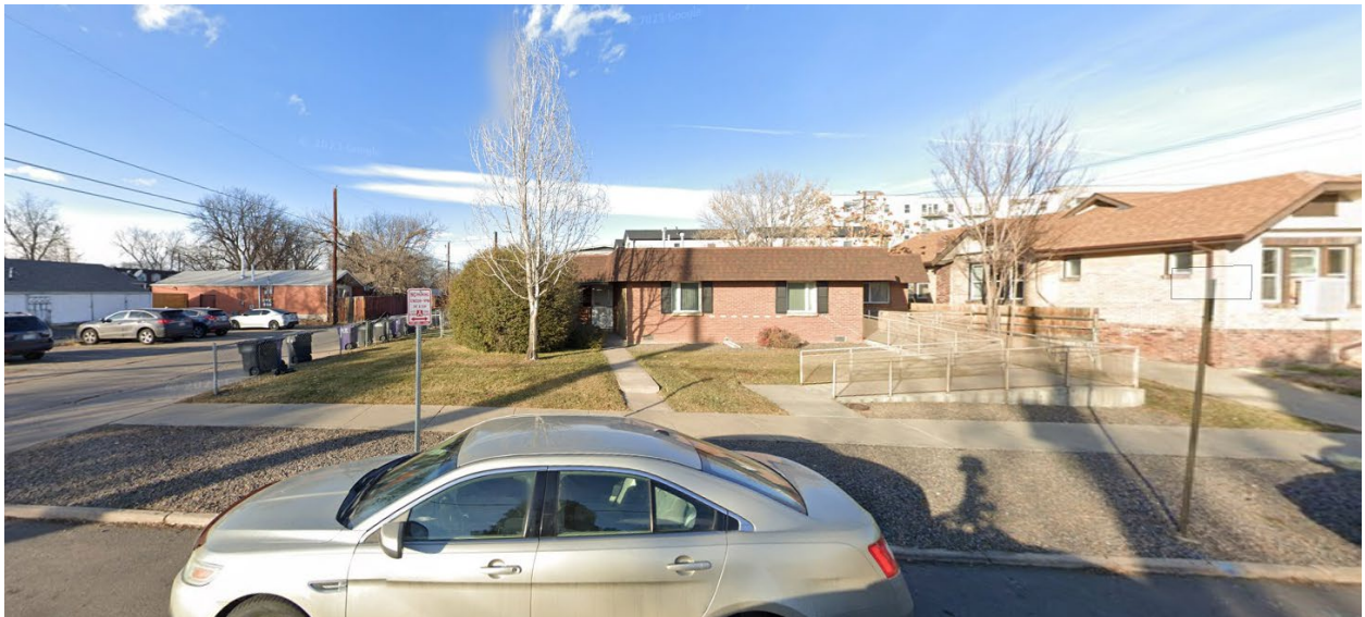
Subject Site (3315-3317 West 14 th Avenue) - View of the subject property, looking North (on West 14 th Avenue)
