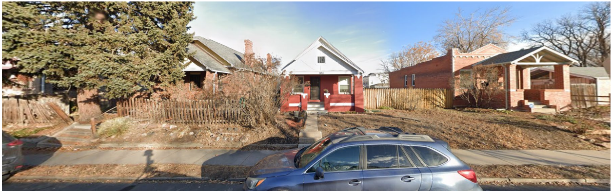
East – View of properties to the East of 1409-1471 North Julian Street (on North Julian Street)
