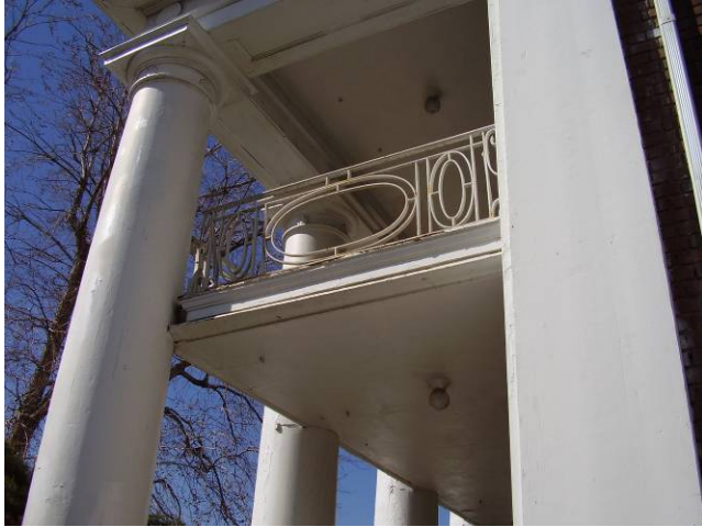
Photo 5 – 2070 Colorado Blvd. columns & porch (2012)
