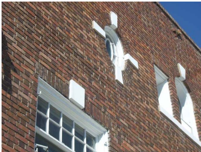
Photo 3 – 2070 Colorado Blvd. window detailing (2012)
