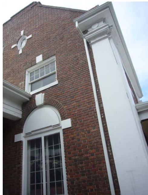
Photo 4 – 2070 Colorado Blvd .pilaster & windows (2012)
