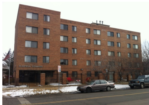
Apartments across Downing Street to the east
