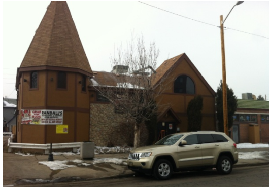
View of subject site from Downing Street
