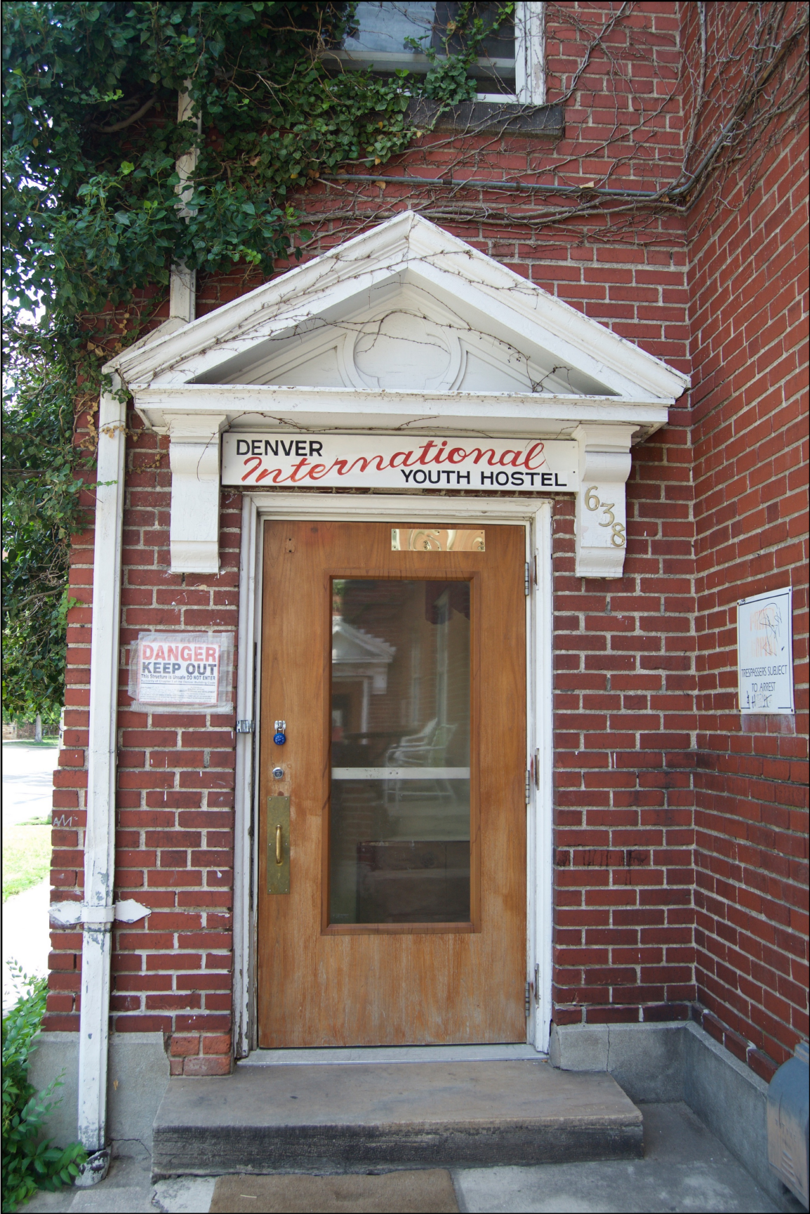
Main entrance into east wing
