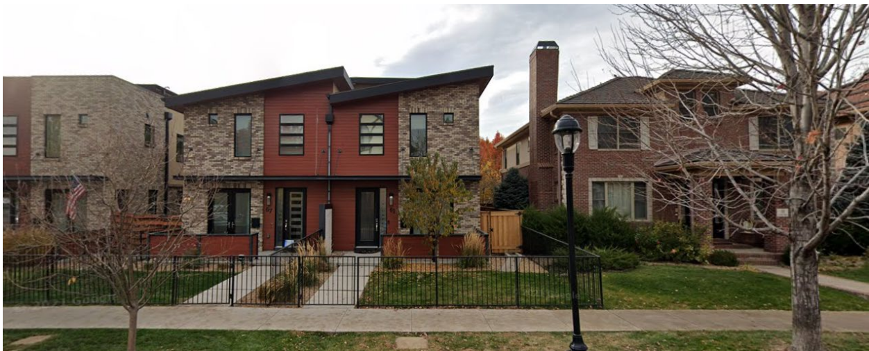
View facing west on Garfield Avenue north of Bayaud Avenue
