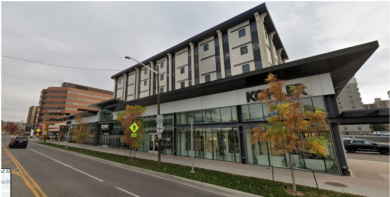
View facing southeast on 1 st Avenue east of Adams Street
