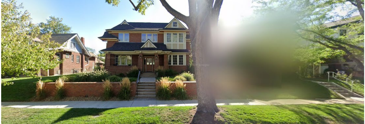
West - View of the properties to the west (across the alley).
