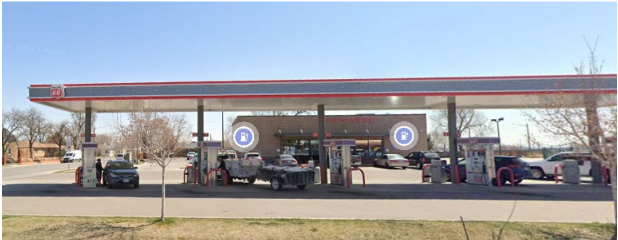
Gas station located directly north of the subject property, facing east from Federal Boulevard.
