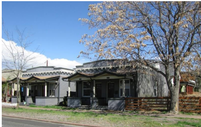
Structures in proposed district, example of Terrace buildings
