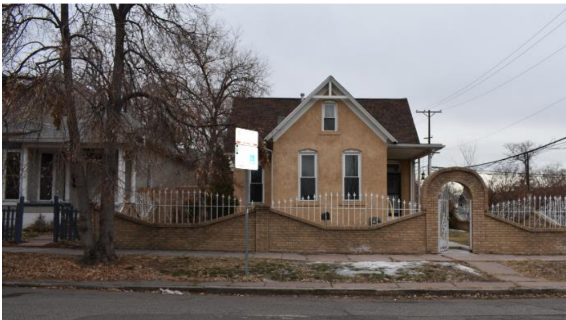
Structure in proposed district (note addition of stucco and fencing)
