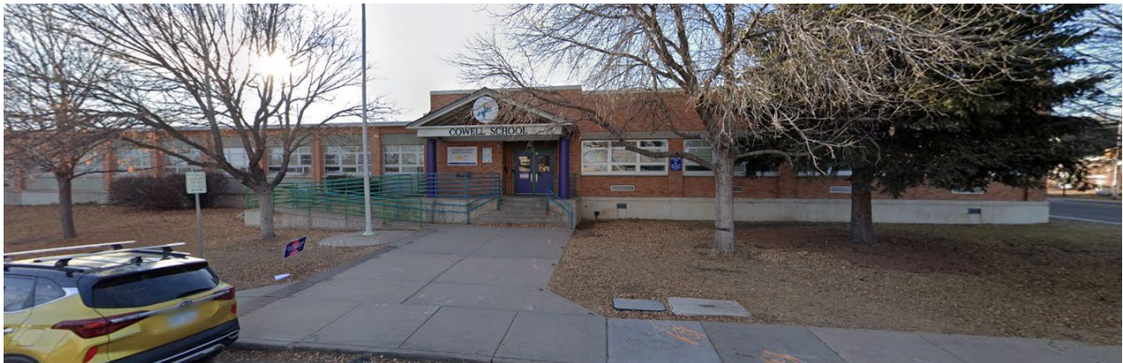
West – Cowell Elementary School, looking west from North Utica Street
