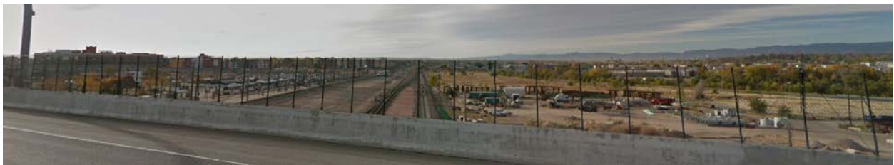
Looking west from Mississippi Avenue showing the rail underpass
