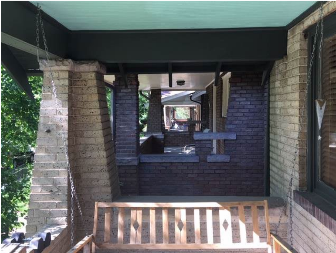
Figure 1 The Bungalow porches present physical and design-based connectivity up and down Steele Street
