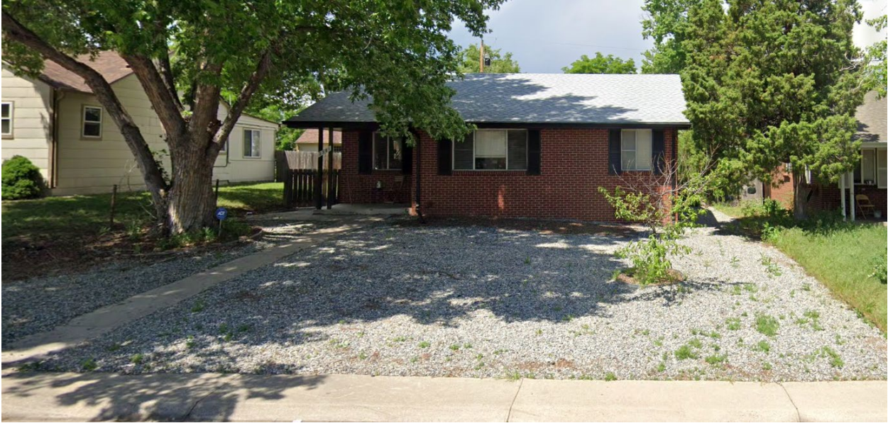
View of the subject property, looking west.
