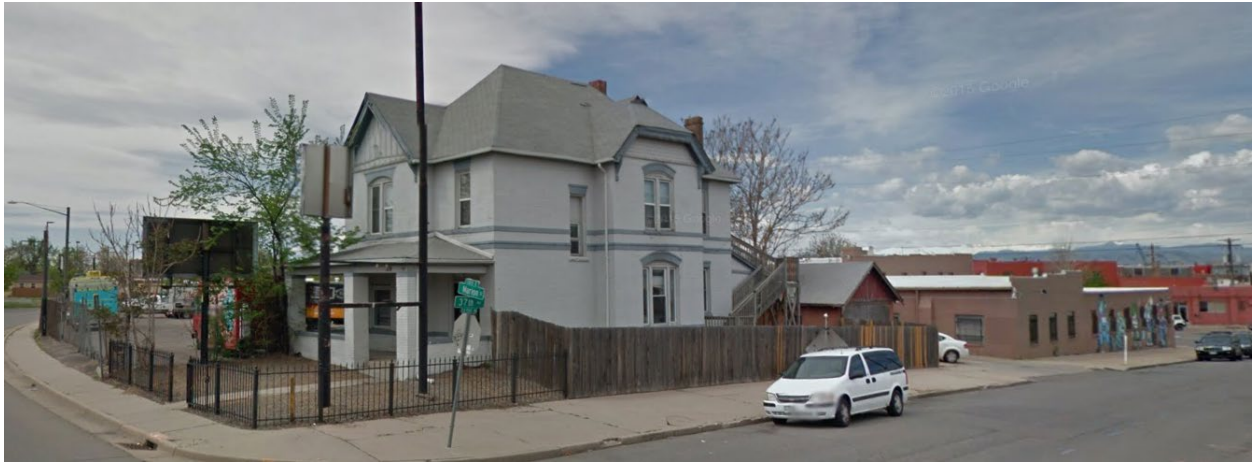
Subject Property Looking West from Marion Street at 36 th Avenue
