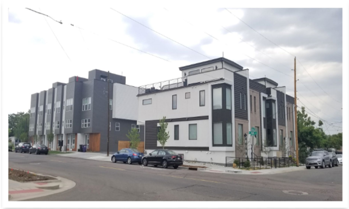
Figure 8: New multi-Unit development at W. 46 th Avenue and Shoshone Street
