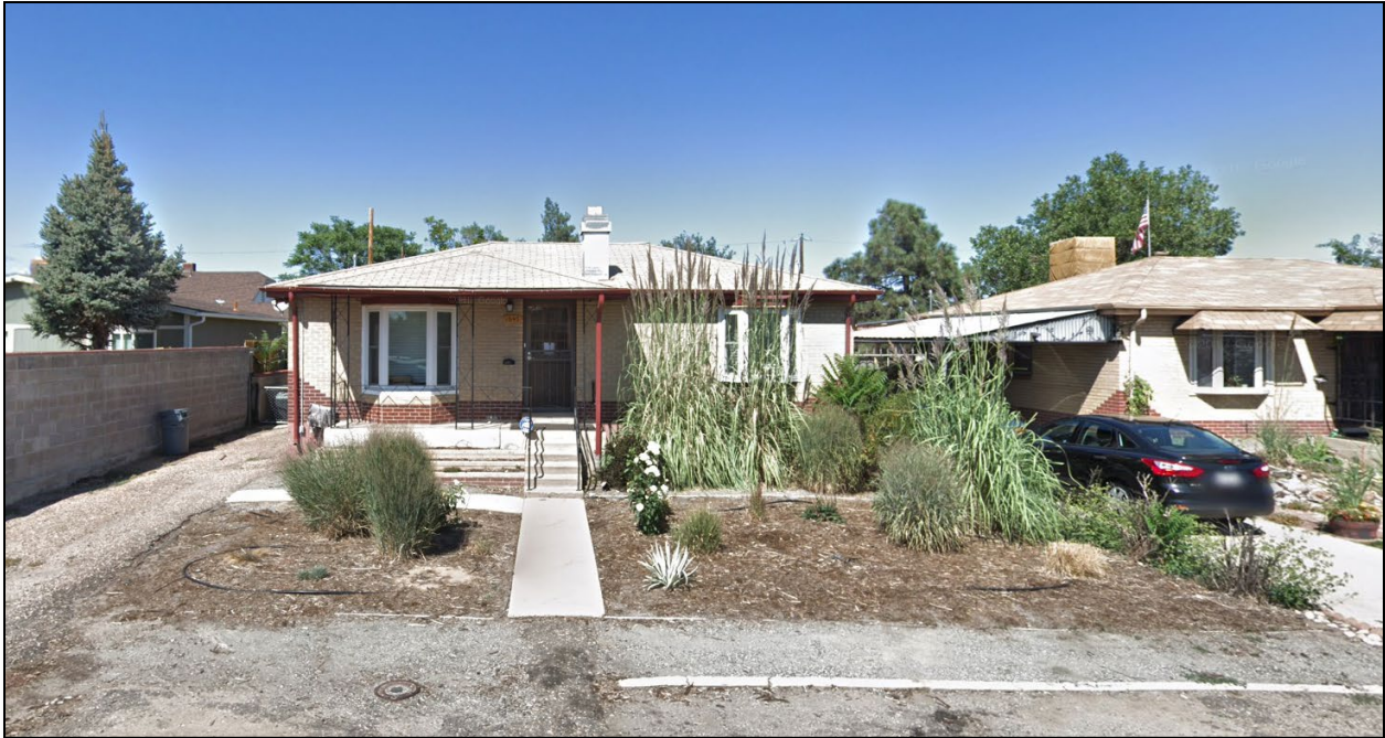
Figure 6b: View of Subject Property from W. 46 th Avenue with single-family home visible to the right
