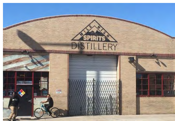
Most older buildings in Arapahoe Square are 1-3 stories in height.
