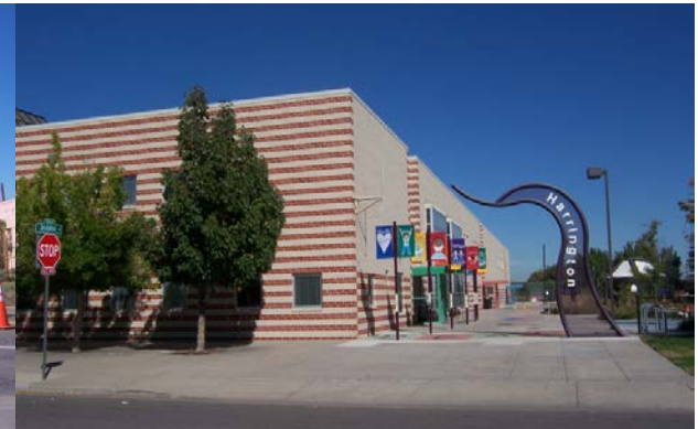
Elementary School east of subject property
