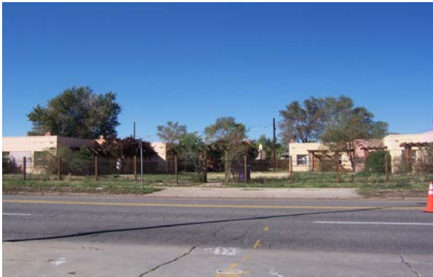
Multi-unit residential west of subject property.
