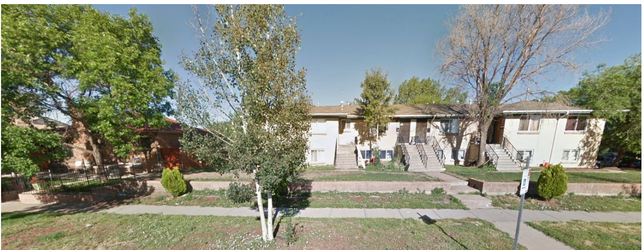
Property to the west of the site on Gaylord Street, looking west.
