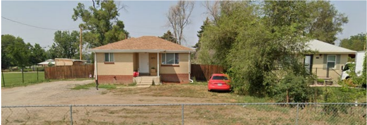
View of the property directly east of the subject site, looking north from W. Kentucky Ave.
