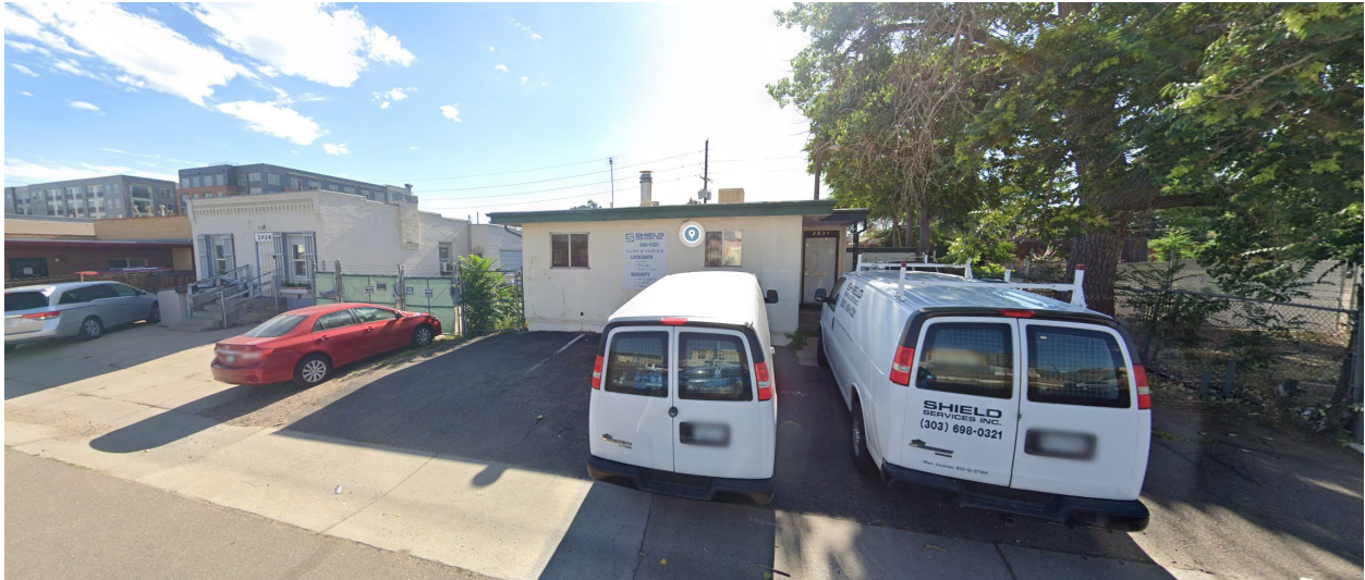
North – from South Bannock Street looking northeast
