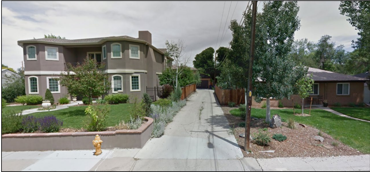
View of properties on Adams St. north of Yale Ave.
