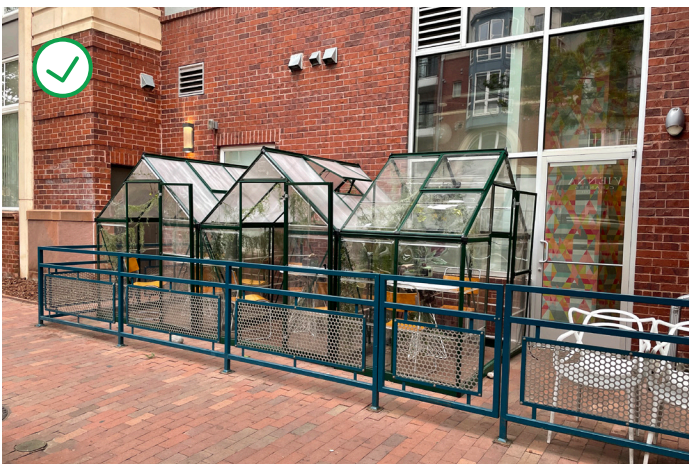
↑ Maximize transparency on all sides of the enclosure to maintain visibility into and through the structure.
