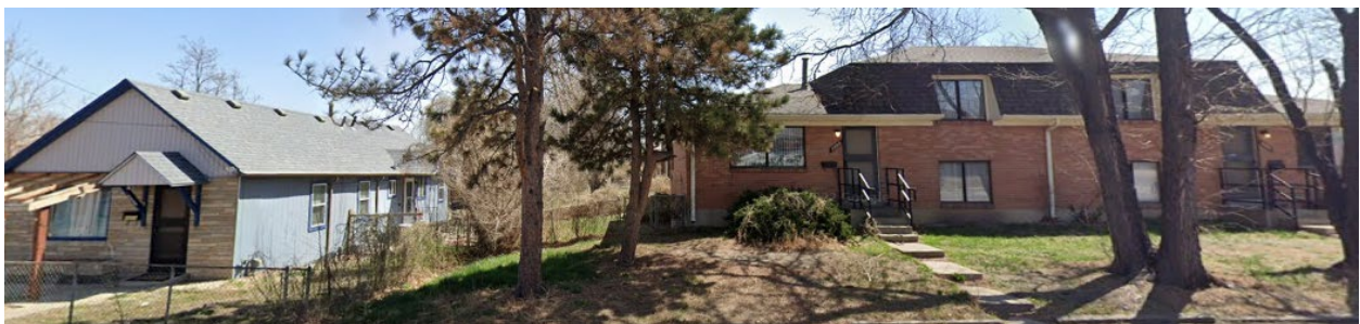
View facing east on Pecos Street between W 44 th and W 46 th Avenues – east of proposed rezoning.
