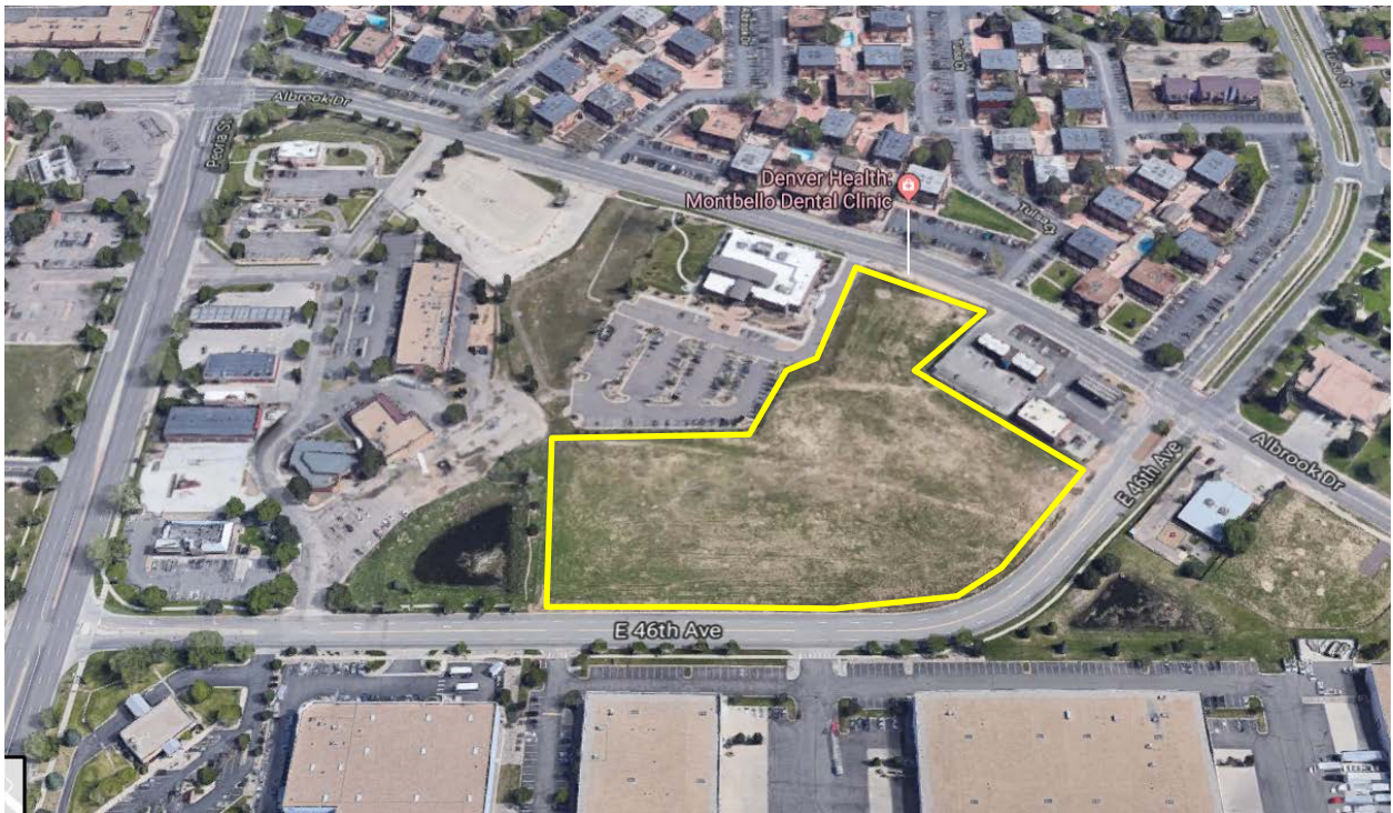
Aerial view of subject site and surrounding properties (source: Google Maps)
