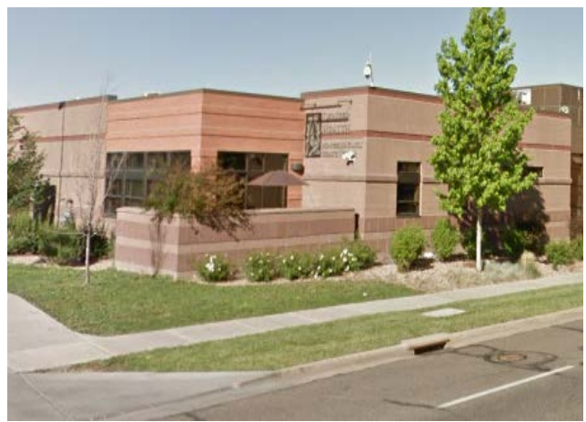
Clinic to the west of subject site. View from Albrook Dr. looking west.
