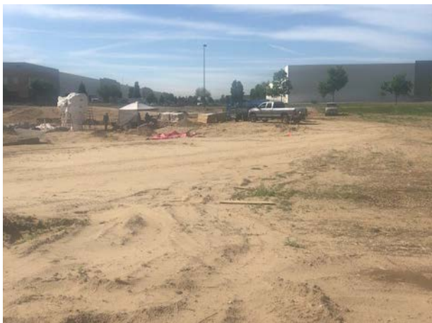
View of site from Albrook Dr. looking south
