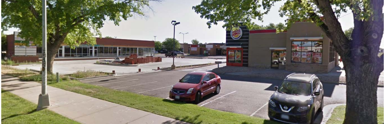
Commercial development to the west of site looking northeast from Peoria St. (source: Google Maps)
