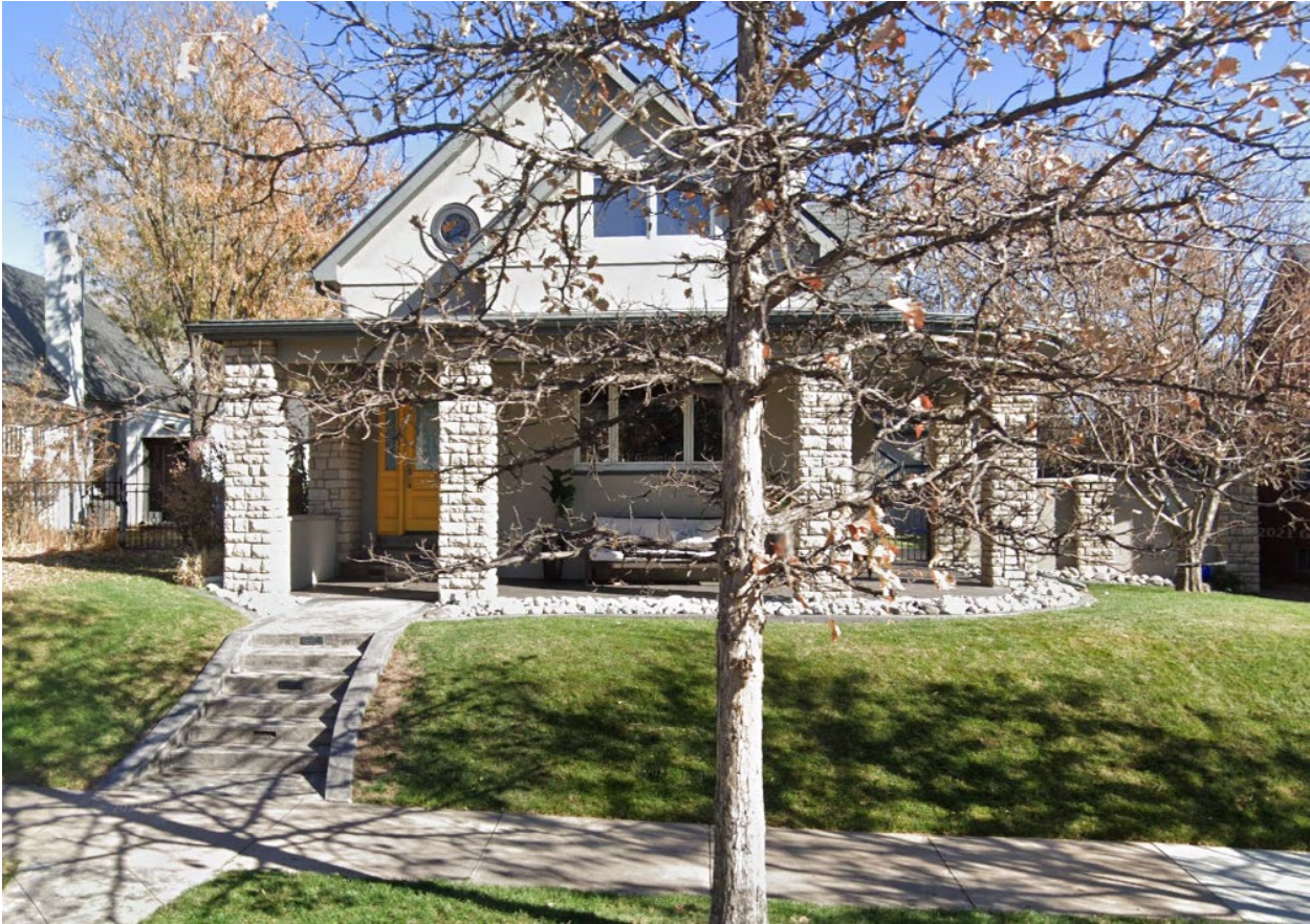
North - View of the property to the north, looking east
