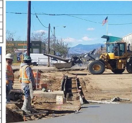
Progress on Brighton Boulevard
