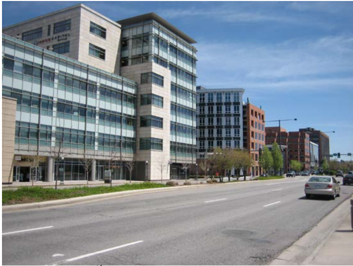
Context along 1 st Avenue
