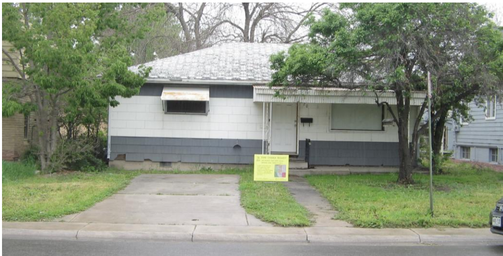
Subject site, looking east from South Madison Street
