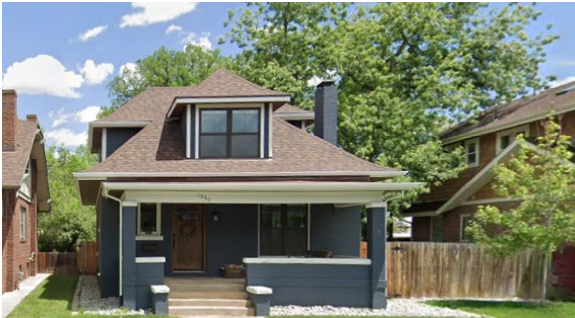
View of subject property looking east.
