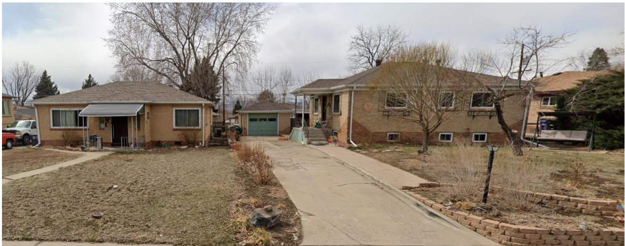
South - View of properties to the south, looking east.
