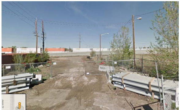
West – BNSF Rail right-of-way corridor.
