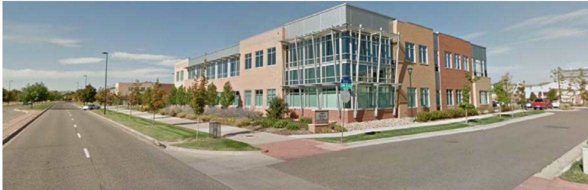
Image source: Google, image date: September 2011
