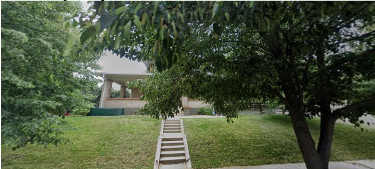
View of subject property along North Hooker Street facing west.
