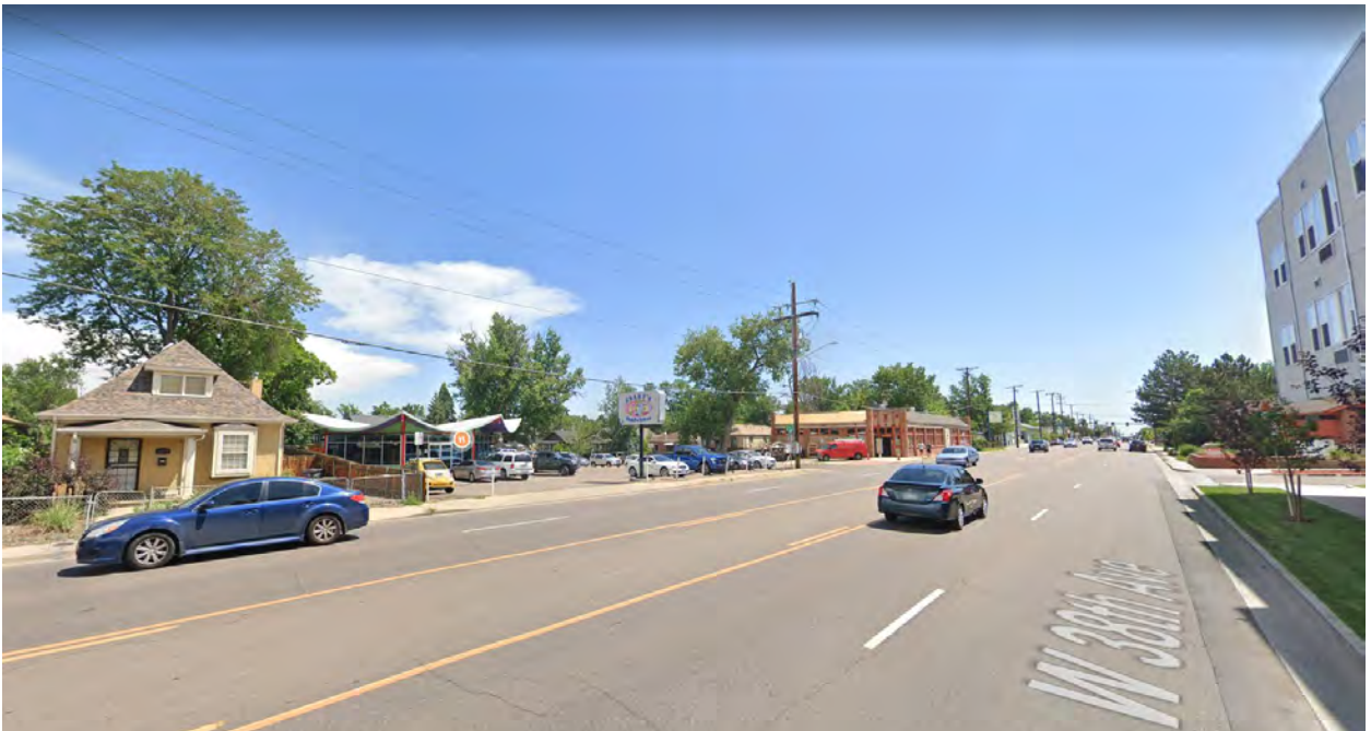
View facing east on 38 th Avenue between Yates Street and Zenobia Street (U-MX-3)
