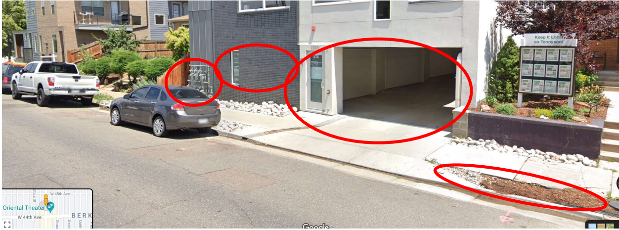
Figure 4 – Pedestrian experience includes a garage entrance, undersized tree lawn, and gas meter bank with a false front door and a single small window looking into a garage.
