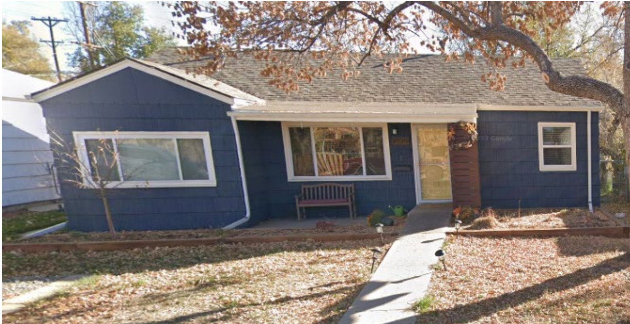
Subject Site - View of the subject property, looking east.
