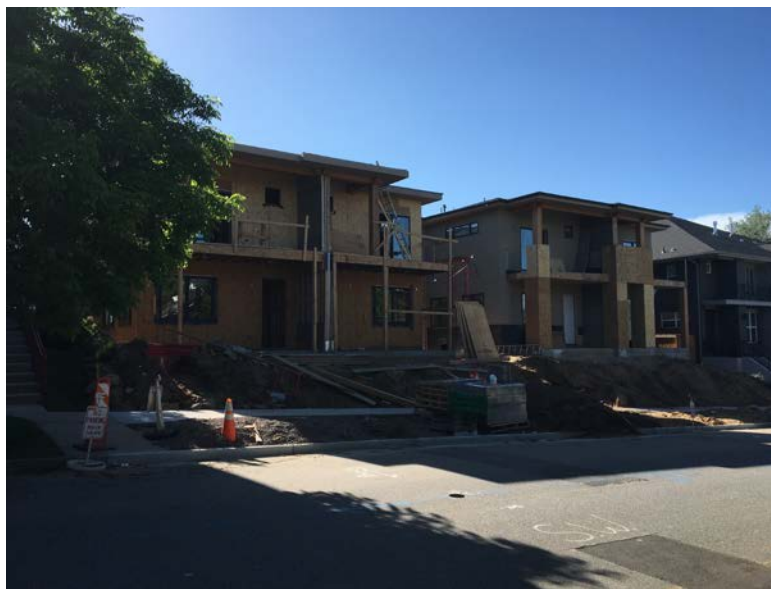
Two duplexes are under construction due west of the subject site, across the alley and facing Jackson Street.
