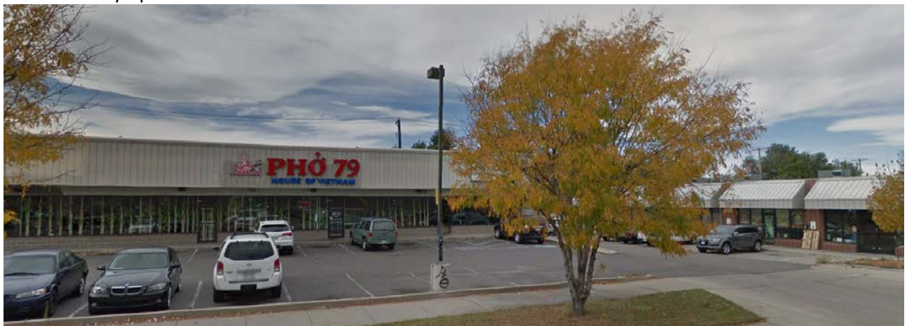
West: 1 story Commercial across Federal Blvd
