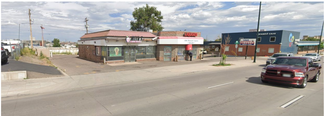
View of the properties to the south of the subject property, looking east from Federal Boulevard.
