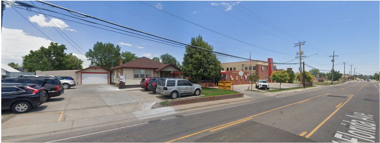
3145, 3151 & 3155 West Florida Avenue - View of the subject properties, looking northeast.
