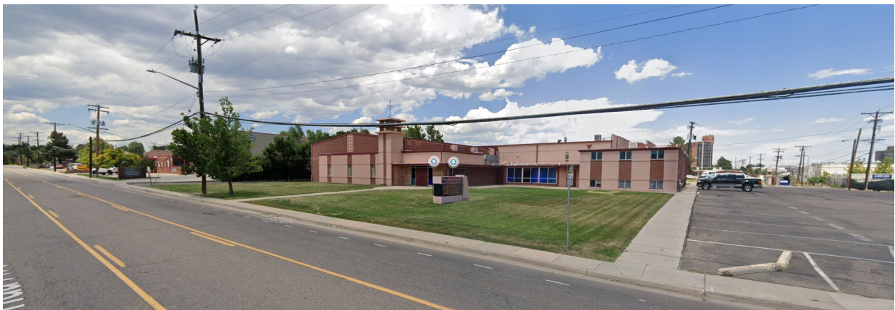
East - View of the church east of the subject site, looking northwest on West Florida Avenue.
