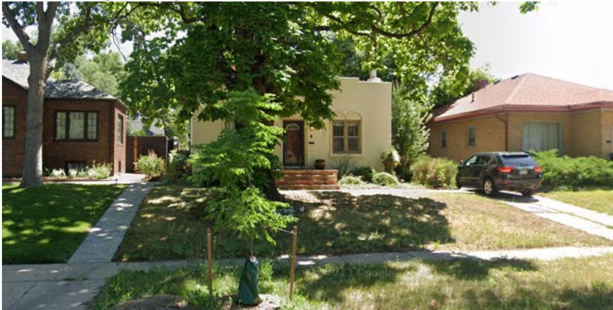
Subject Site - View of the subject property, looking east.
