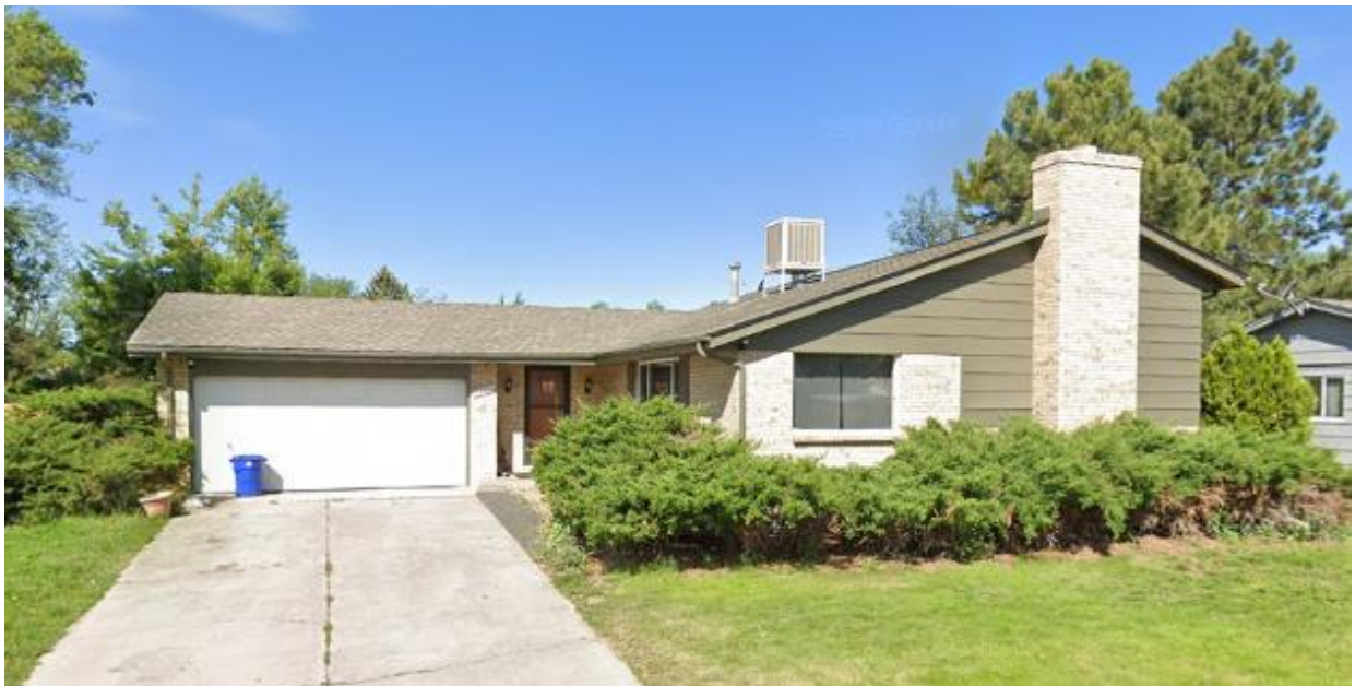
View of the property to the north, looking west.
