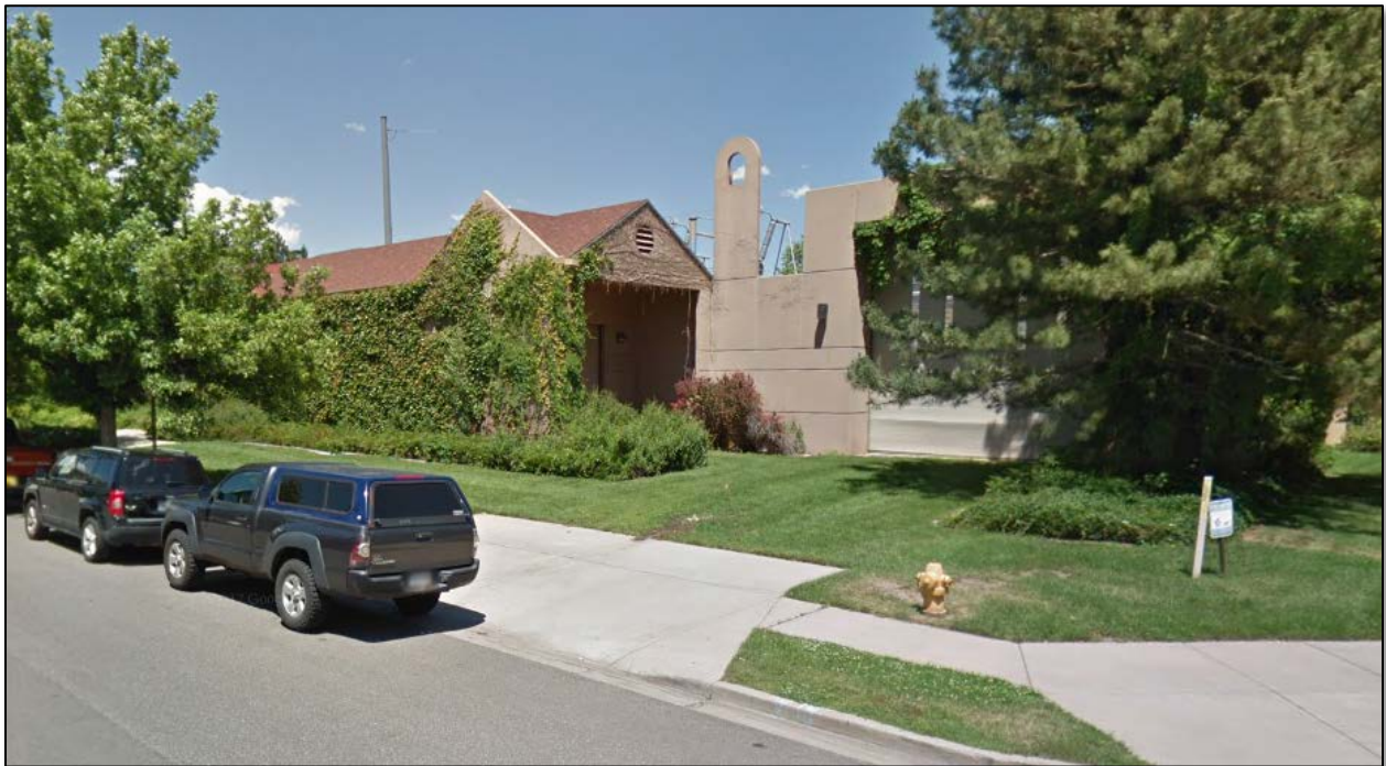
Figure 6e: View of Xcel Substation to the South
