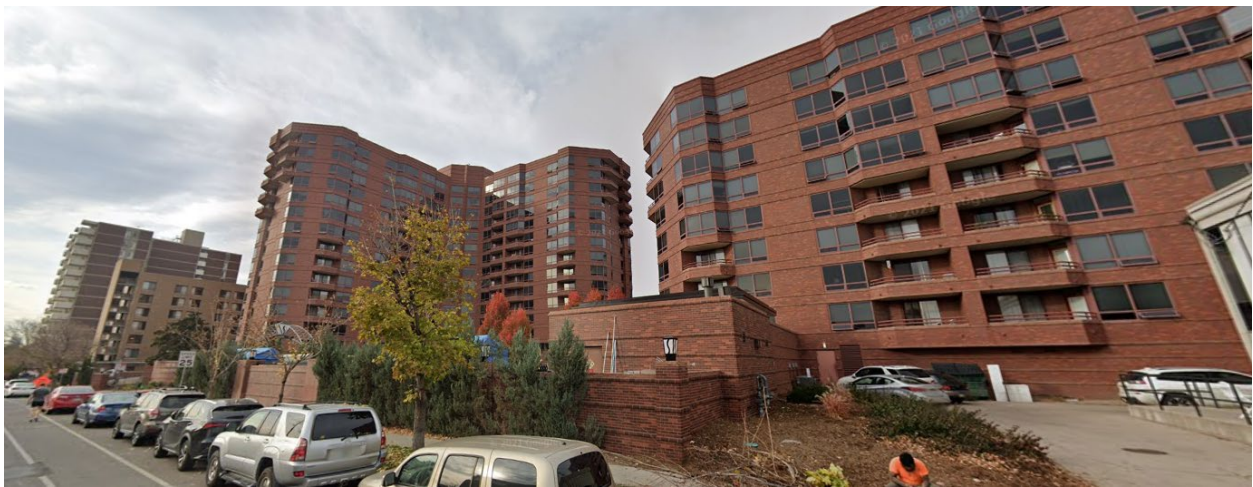
North - Looking northwest from E. Bayaud Ave.
