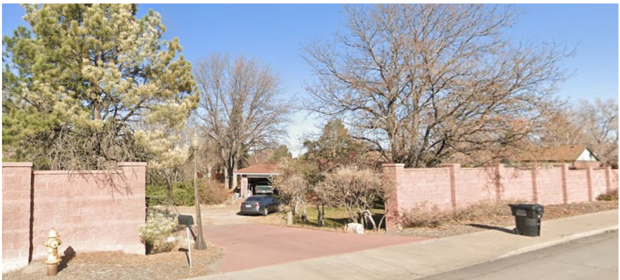
View of the property to the east looking north from Mississippi Ave.
