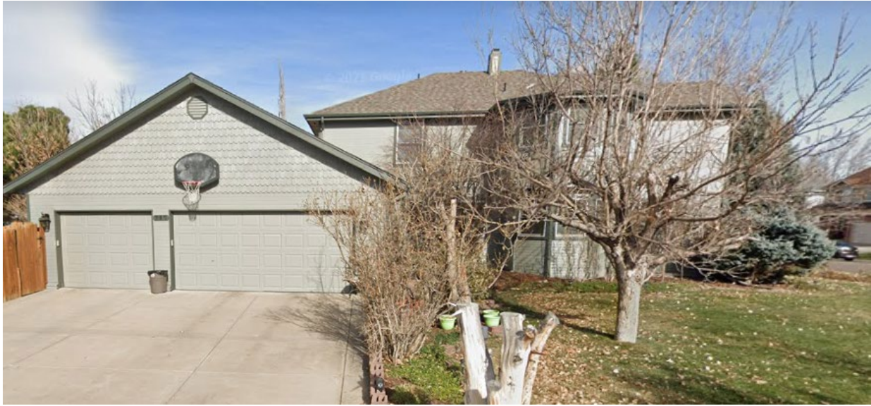
View of the property to the north, looking north.
